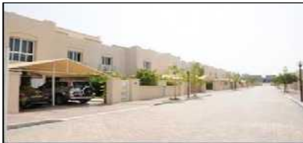
17 Villa complex at Azaiba - MEP Works
