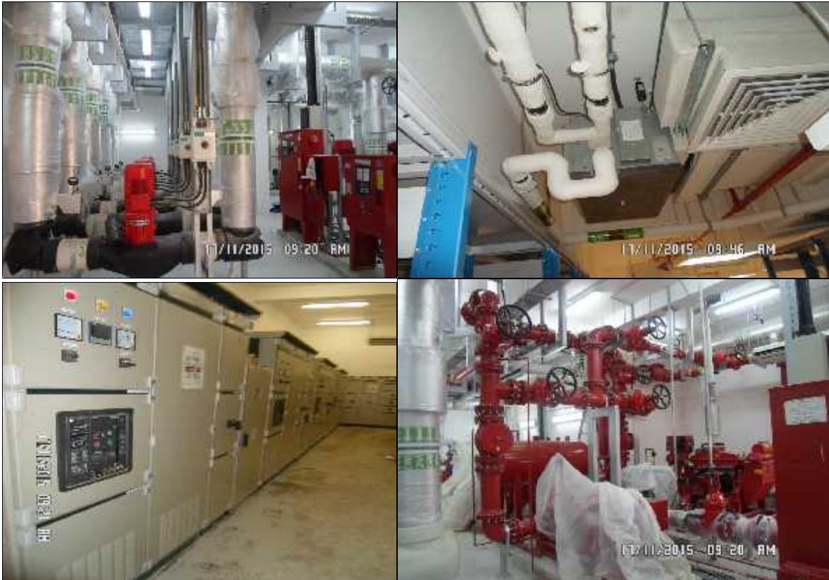
Supreme Court at Al Ghubrah - MEP Installations
