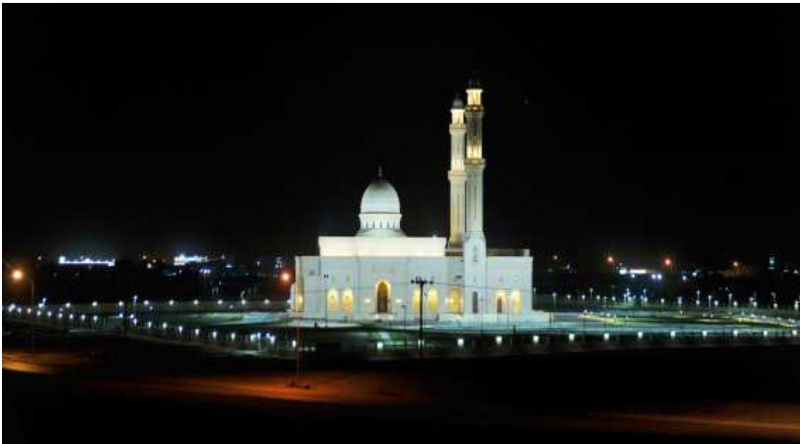
Sultan Qaboos Mosque at Bu Ali – MEP Works
