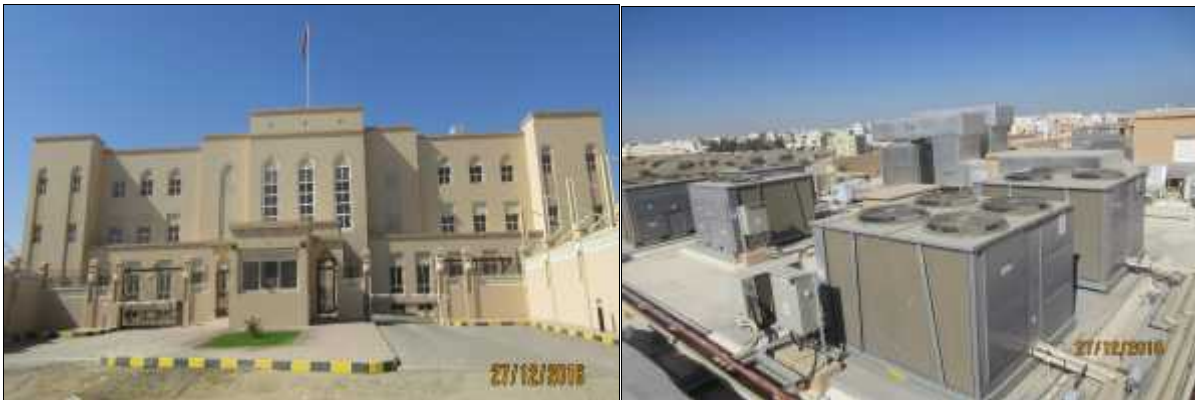
Offices for DG of General Affairs at Mawaleh – HVAC Installations
