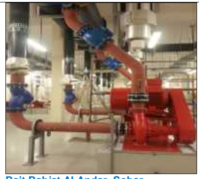
Bait Bahjat Al Andar, Sohar – Infrastructure Development works
