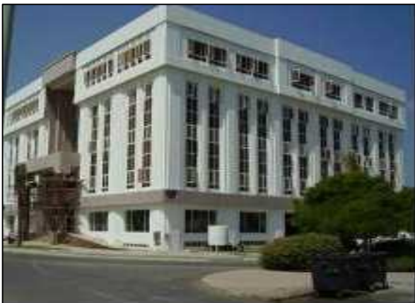
Commercial Complex at Shati Al Qurum - Electrical and Plumbing works.
