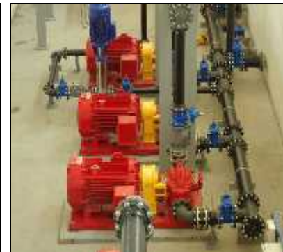
Plumbing Installations at Sohar Airport- Package-1 & 2
