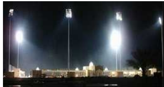
New Parade Ground at Shafa – Highmast Installations for MOD
