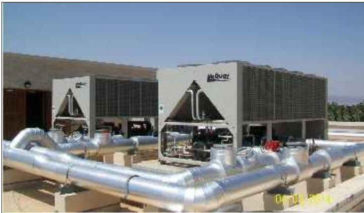
RCA Office Bldg. at Nuwedra, Salah MEP Works
