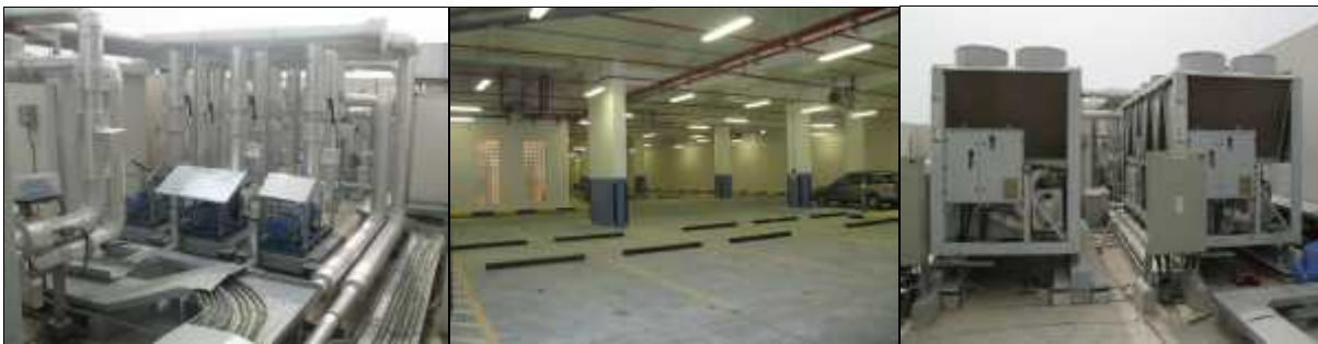
Qalhat LNG Head Quarter Building at Ghala - MEP Installations
